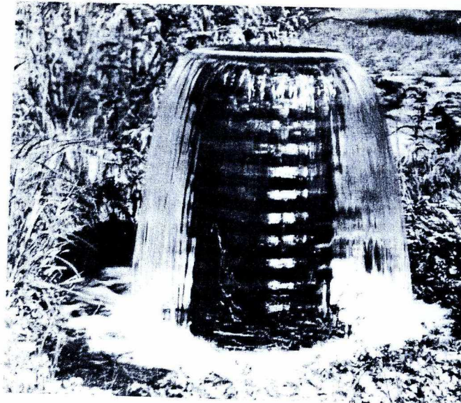
(above) Figure 12. Toe drain outlet in dam-site area.
