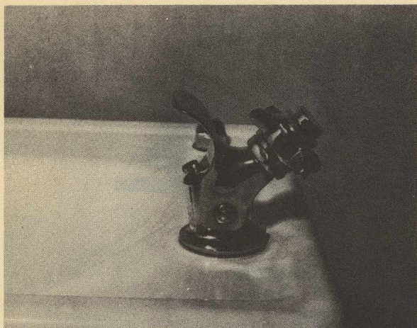
(5) The nozzle should be above the edge of the bowl so that dirty water in a flooded bowl will not cover the nozzle.
