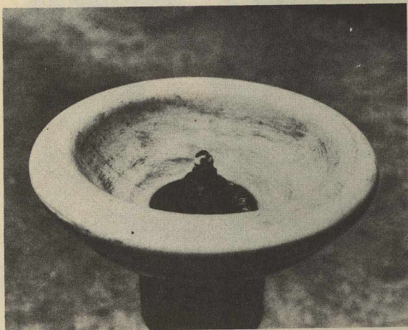
(1) This improperly designed drinking fountain may transmit disease.
