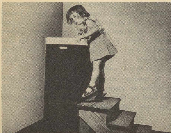
(9) LEFT: Persons of any height should be able to reach the jet. Steps should be provided for children.
