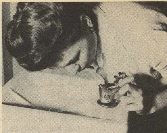
(6) The nozzle should be protected by a guard to prevent dripping water and the user's lips from reaching it.
