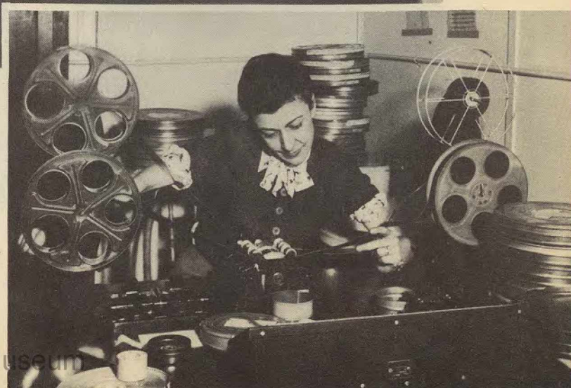
Sound and film are on separate negatives. The editor synchronizes the two negatives.
