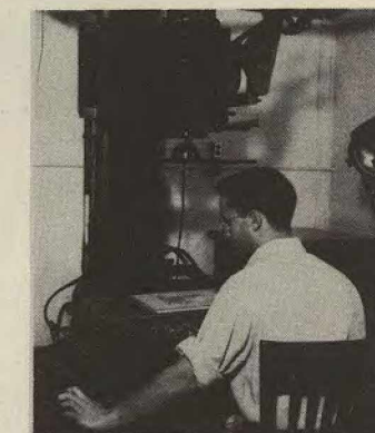
The animation stand is used for shooting titles, charts, maps, and animation.
