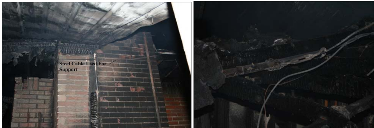
Photo 1. Steel cable used to support the chimney against the house with a turnbuckle. (Photos courtesy of sheriff's office)
