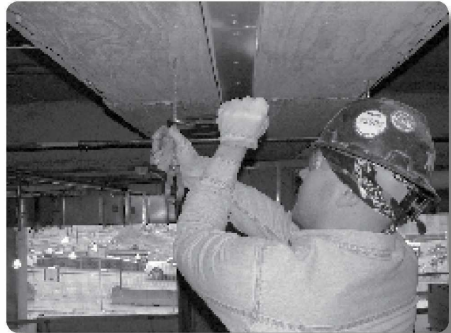
Problem: Tightening conventional nut on all-thread
