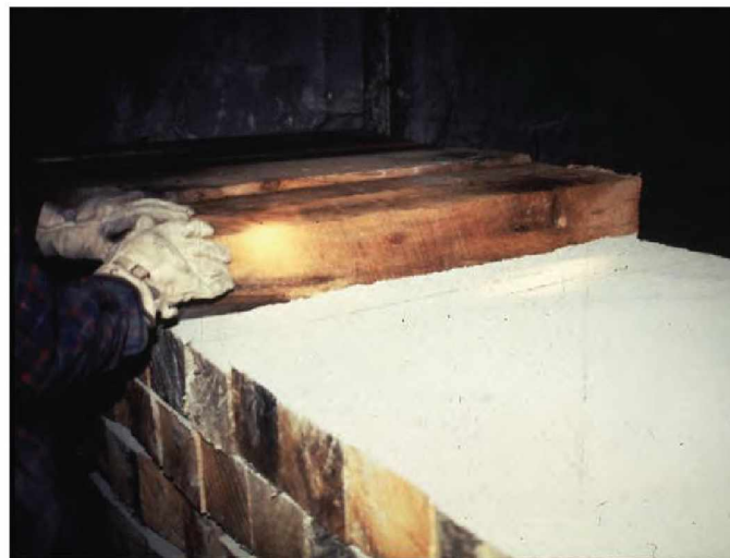
Figure 39.—Closeup of a hitched wood-crib-block seal showing the layer of rock dust placed between each layer of wood crib blocks.
