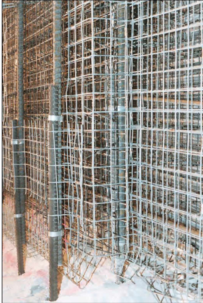
Figure 19.— Insteel 3-D seal under construction with the addition of the front Insteel panel and the front plane of vertical #8 steel reinforcement bars.
