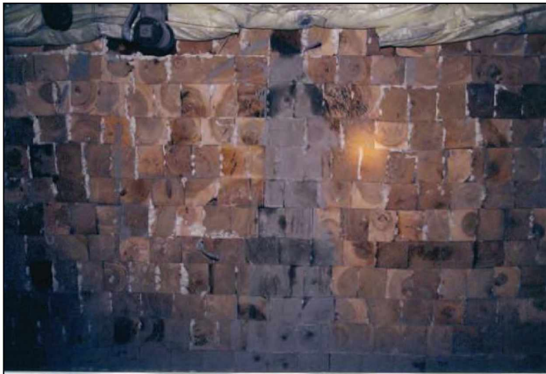
Figure 43.—Construction of a wood-crib-block seal with pressurized Packsetter grout bags in lieu of hitching showing the glued wood crib blocks and the grout bags used along the roof and ribs. The active-mine-side surface is later covered with brattice and coated with an approved sealant.
