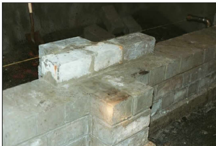
Figure 27.—Solid-concrete-block seal under construction showing the center pilaster and the fully mortared joints on all sides.
