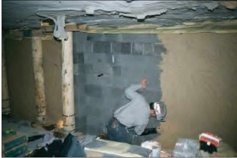
Figure 31.—Tongue-and-groove, solid-concrete-block seal with center pilaster using pressurized Packsetter grout bags in lieu of hitching around the seal perimeter. The worker is coating the seal with an approved sealant.
