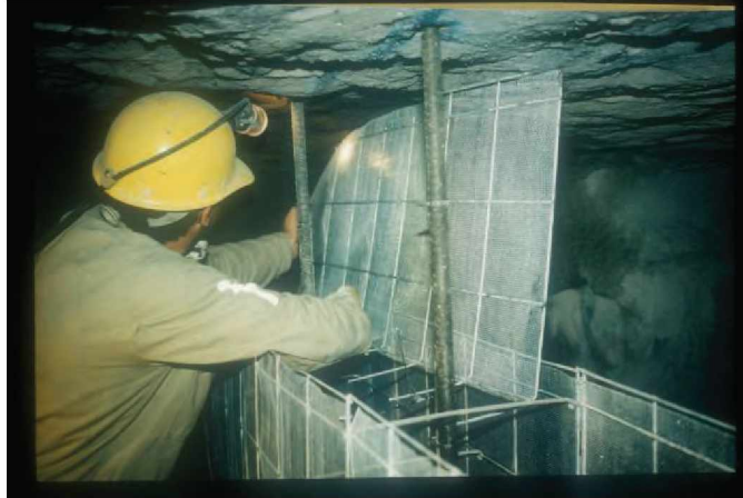
Figure 21.—Closeup of Meshblock seal under construction showing the Meshblocks and the vertical #8 steel reinforcement bars and anchors.
