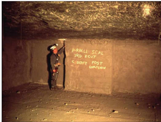
Figure 47.—Completed 24-in-thick Omega block seal showing the angle iron hitch along the ribs and floor and the outer surface coated with an approved sealant.
