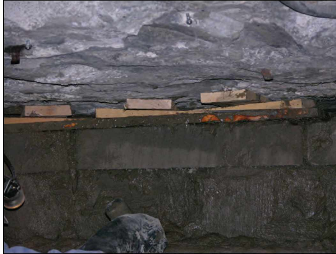
Figure 46.—Construction of an Omega block seal showing the wood board and wedges used to secure the seal at the roof.
