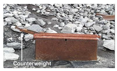
Figure 26.—Counterweight installed to facilitate opening of vault.
