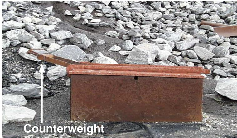
Figure 26.—Counterweight installed to facilitate opening of vault.
