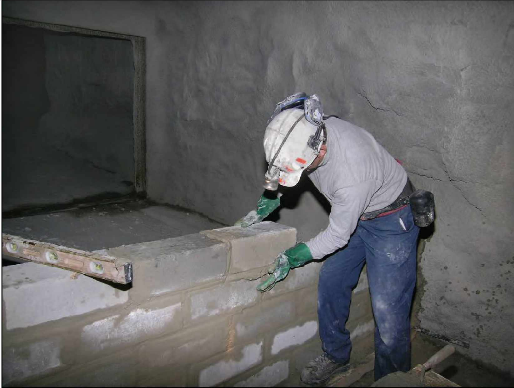
Figure 12.—Wet-laid solid-concrete-block stopping construction with staggered joints.
