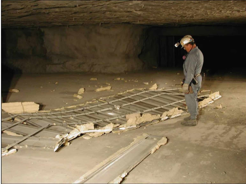
Figure 63.—Debris from steel panel stopping in X-6 after LLEM test #458, viewed from C-drift.
