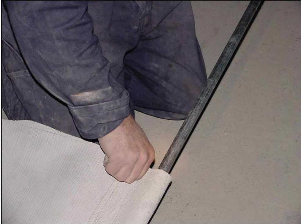
Figure 25.—Inserting pipe into top sleeve of woven cloth.
