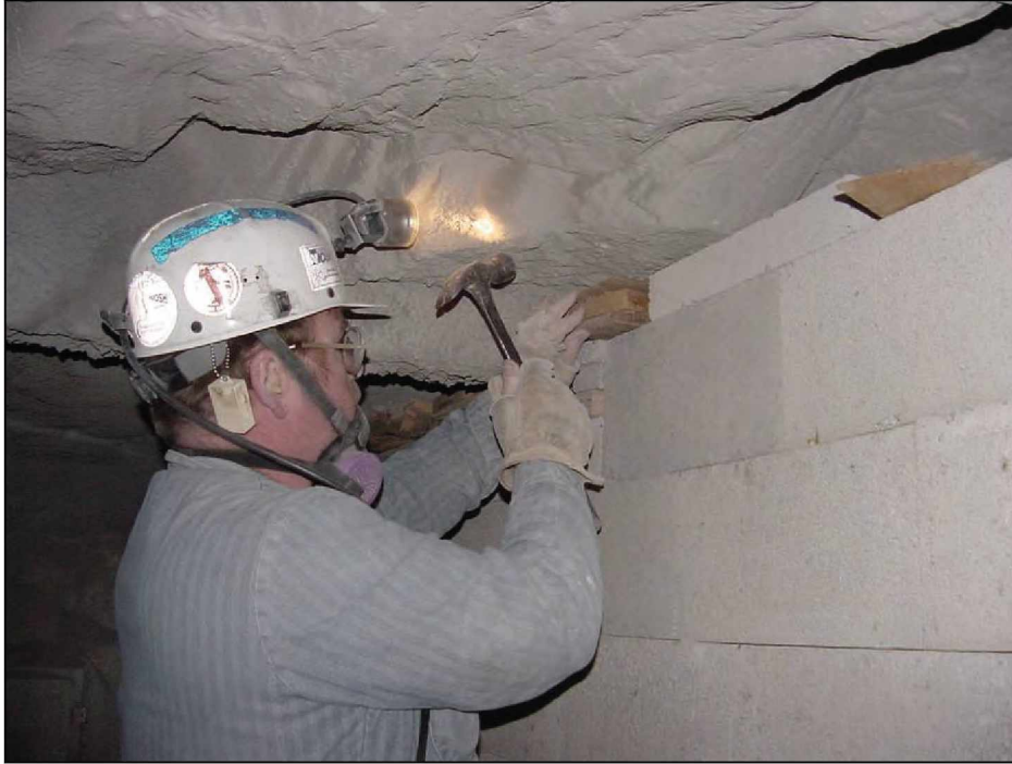
Figure 6.—Installation of wood header boards and wood wedges between the stopping and roof for dry-stacked hollow-core concrete block stopping.
