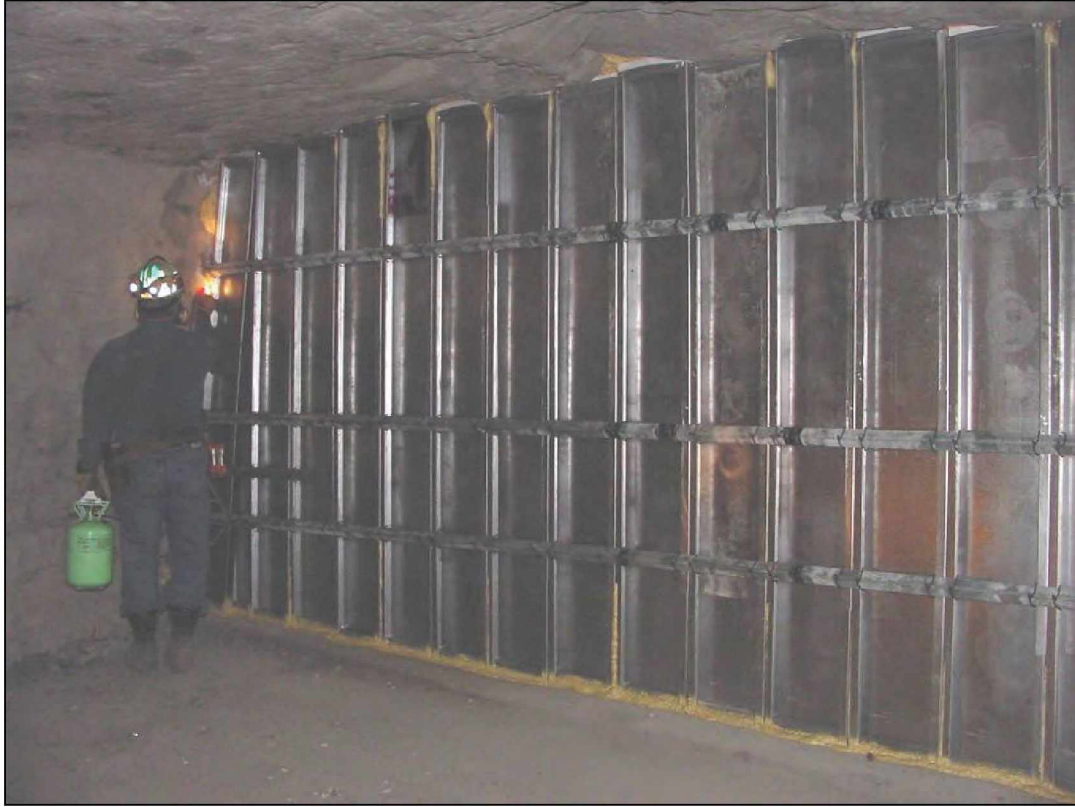
Figure 24.—Nearly completed steel panel stopping in X-6 showing the open panel side attached to the horizontal rib-to-rib angles on the B-drift side.
