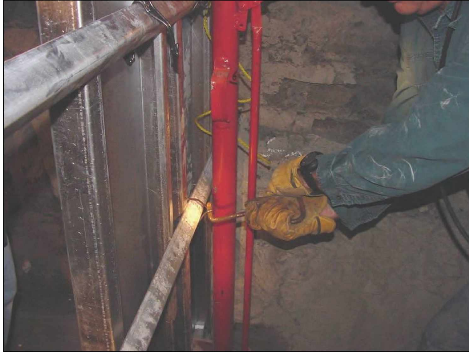
Figure 16.—Horizontal steel angles (with open sides facing panels on left), as viewed from B-drift.
