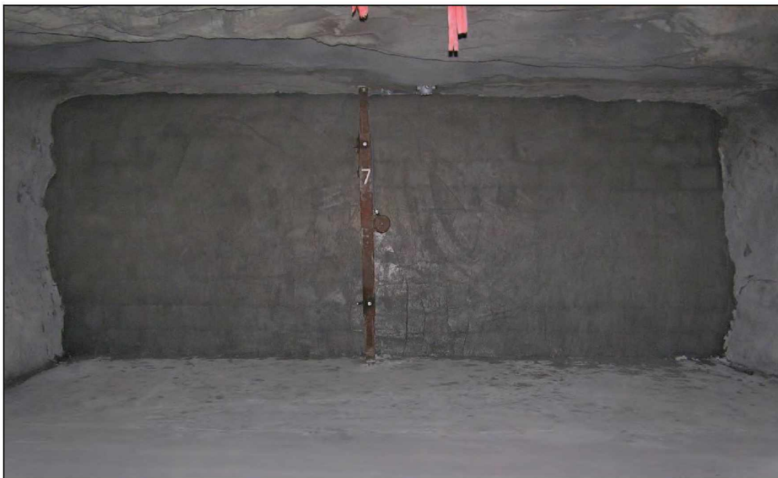
Figure 13.—Completed 6-in (15-cm) thick, wet-laid solid-concrete-block stopping in X-7, as viewed from A-drift.
