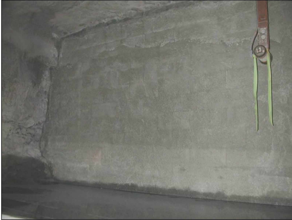
Figure 11.—Completed dry-stacked solid-concrete-block stopping in X-5 as viewed from C-drift, with the total explosion pressure transducer at the upper right.
