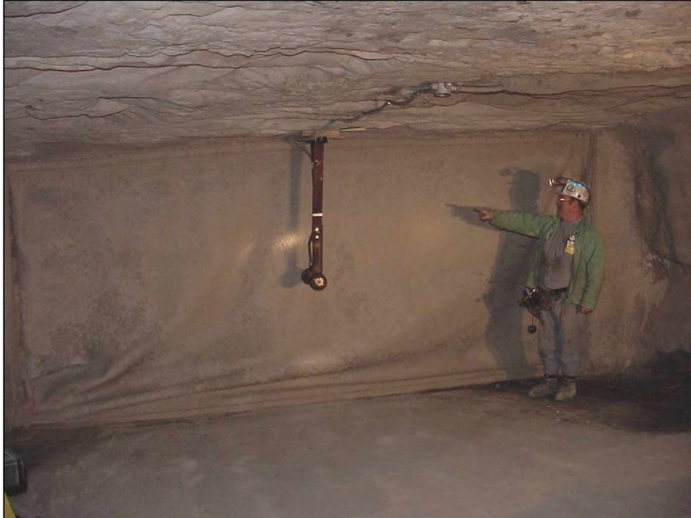
Figure 31.—Completed woven cloth stopping design in X-6, viewed from the explosion or C-drift side.
