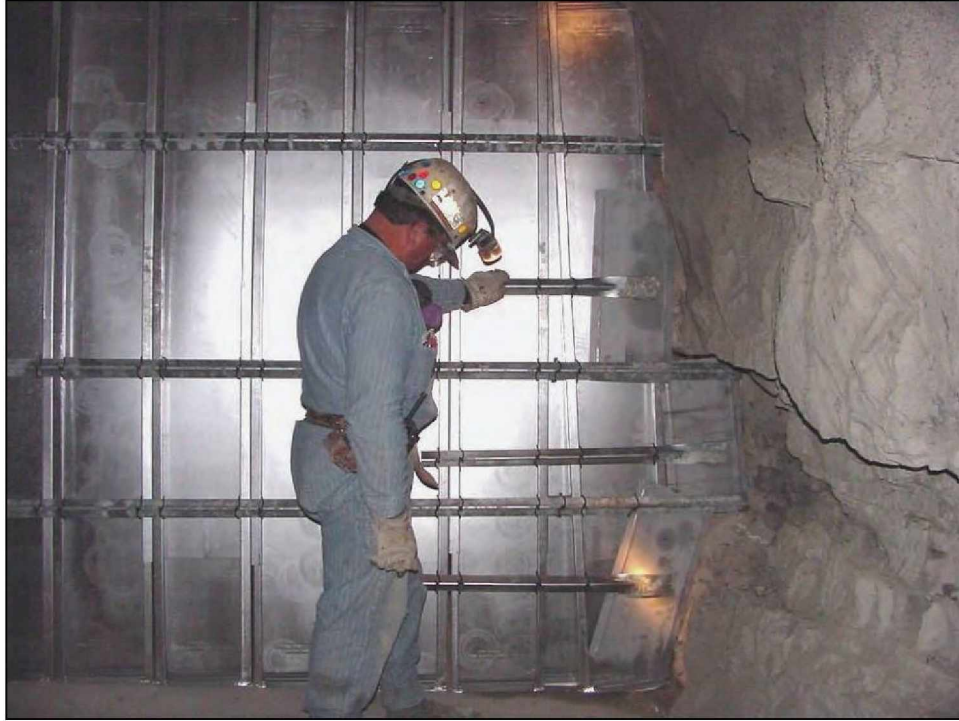
Figure 21.—Side extensions used to fill gaps between rib panel and rib, viewed from the back or B-drift side.
