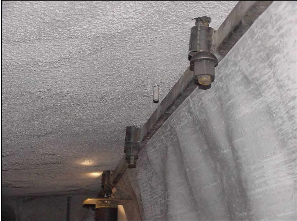
Figure 27.—Anchoring top box section to the mine roof.
