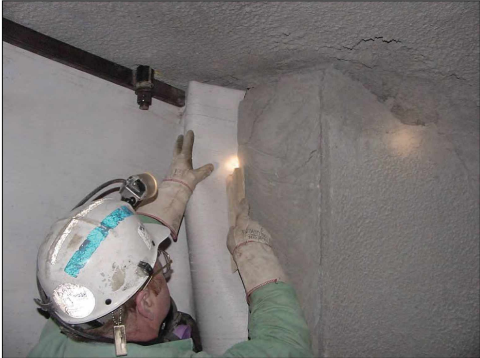
Figure 28.—Wedging woven cloth into mine rib.
