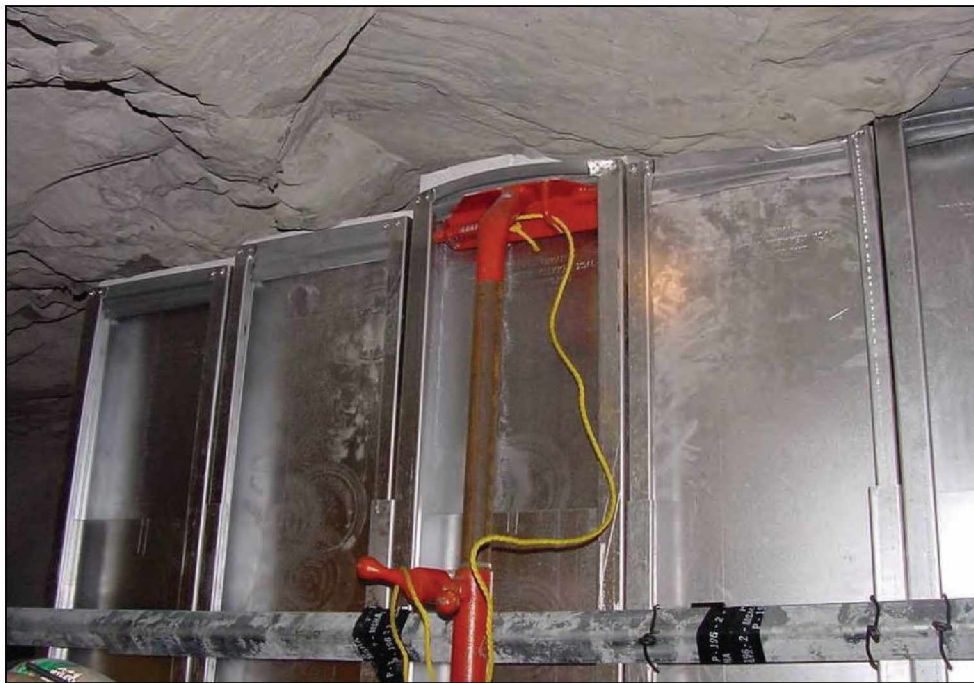
Figure 18.—Temporary jack used to exert roof-to-floor pressure on the metal panel during installation.
