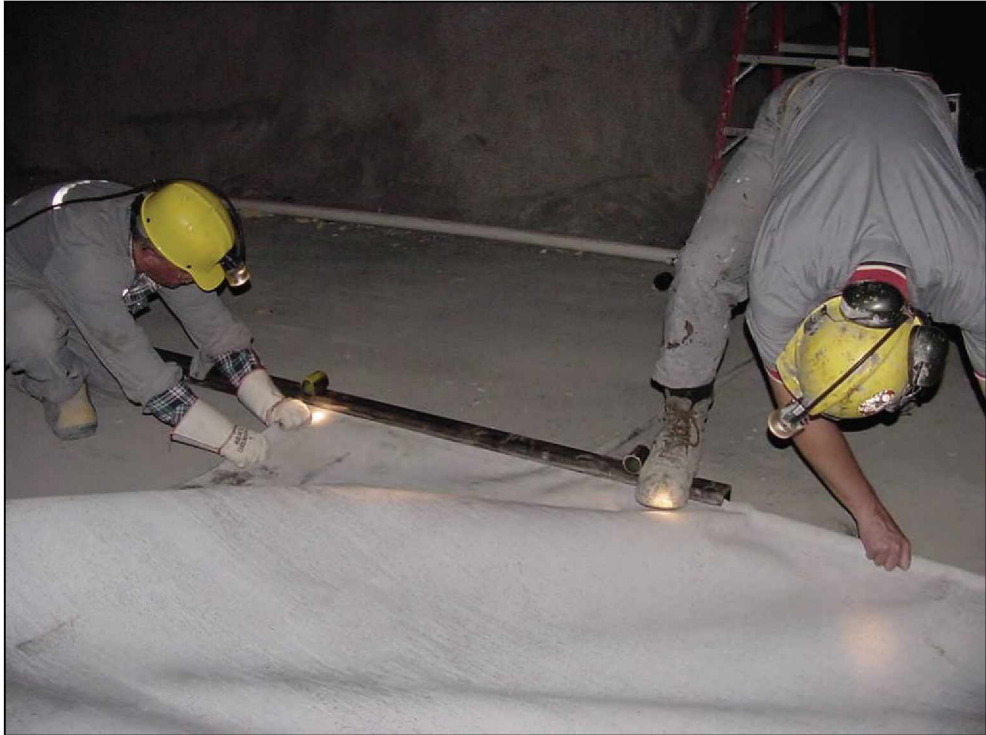
Figure 26.—Inserting pipe/sleeve into top box section.
