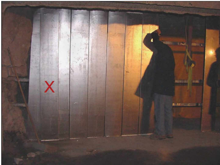
Figure 20.—Overlap panel (indicated by an "X") used to close gap between rib panel and second panel, as viewed from the front or C-drift side.
