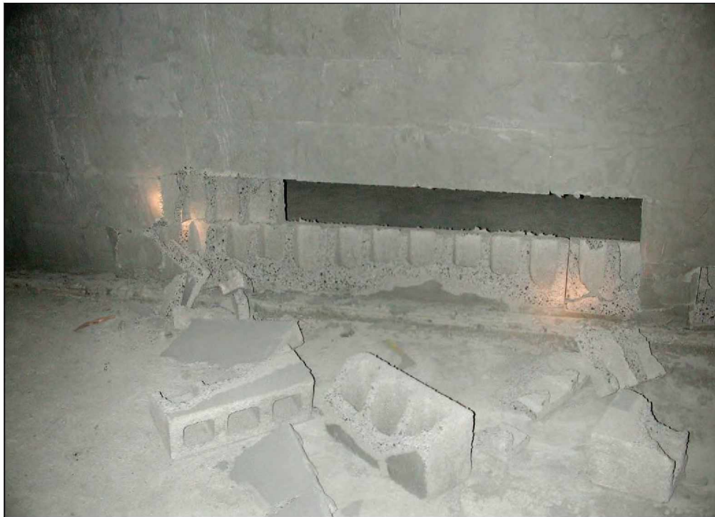
Figure 46.—Closeup of B-drift side of X-6 dry-stacked hollow-core concrete block stopping after test #430, showing dislodged and damaged blocks. This is clear evidence of roof-to-floor arching action.
