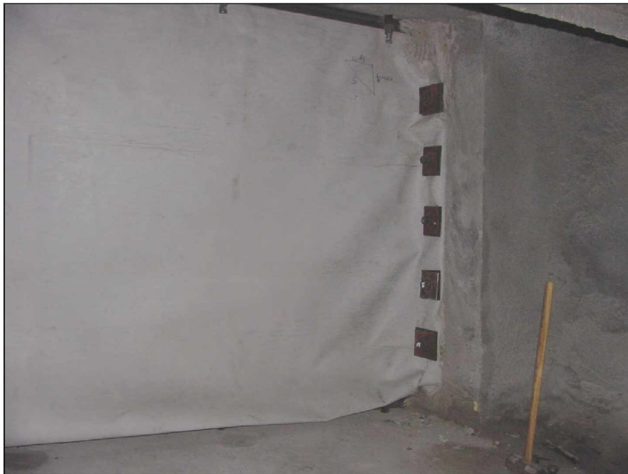
Figure 30.—Rib bolts installed in the X-6 stopping, viewed from B-drift.
