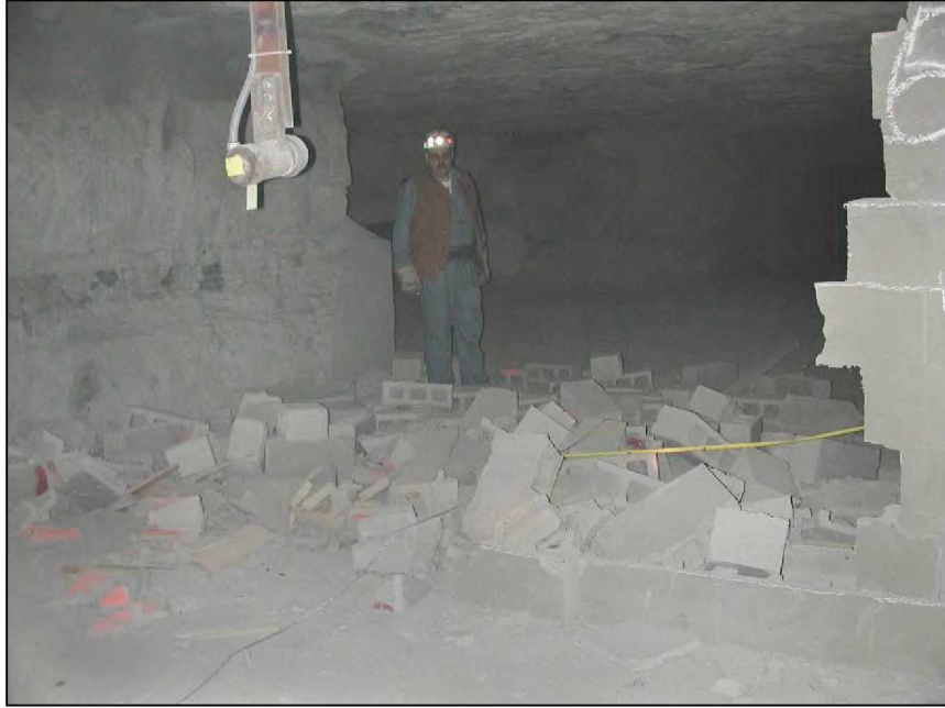
Figure 50.—Debris from X-6 dry-stacked hollow-core concrete block stopping after LLEM test #433, viewed from C-drift.
