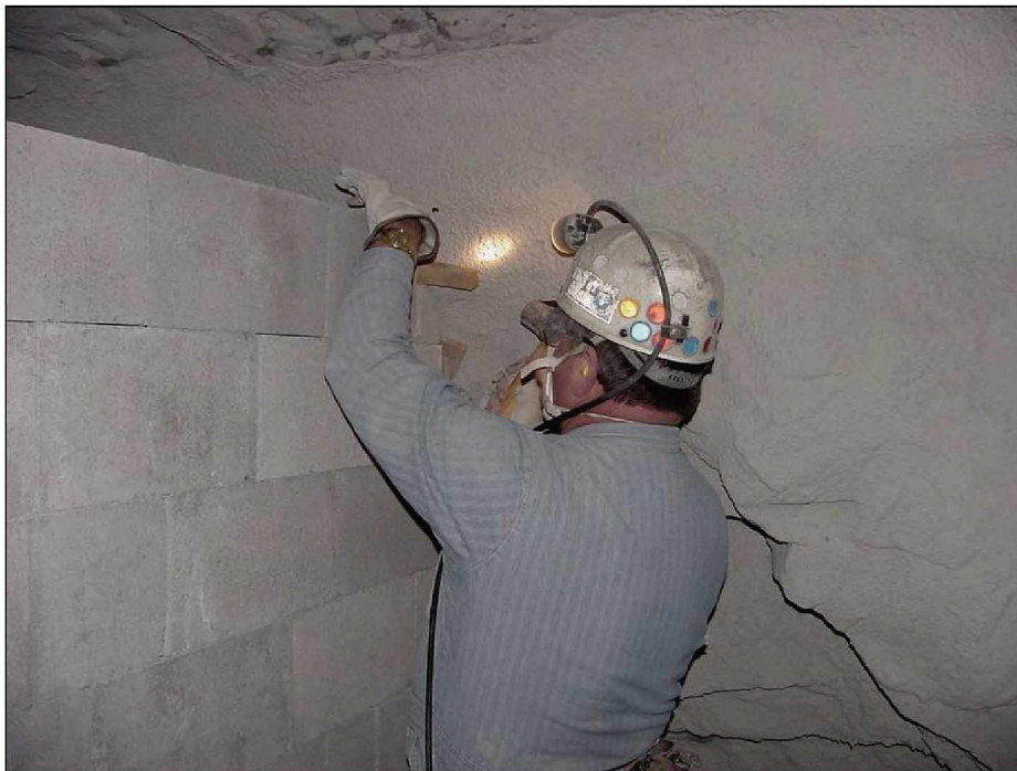
Figure 5.—Installation of wood wedges between the stopping and rib for dry-stacked hollow-core concrete block stopping.
