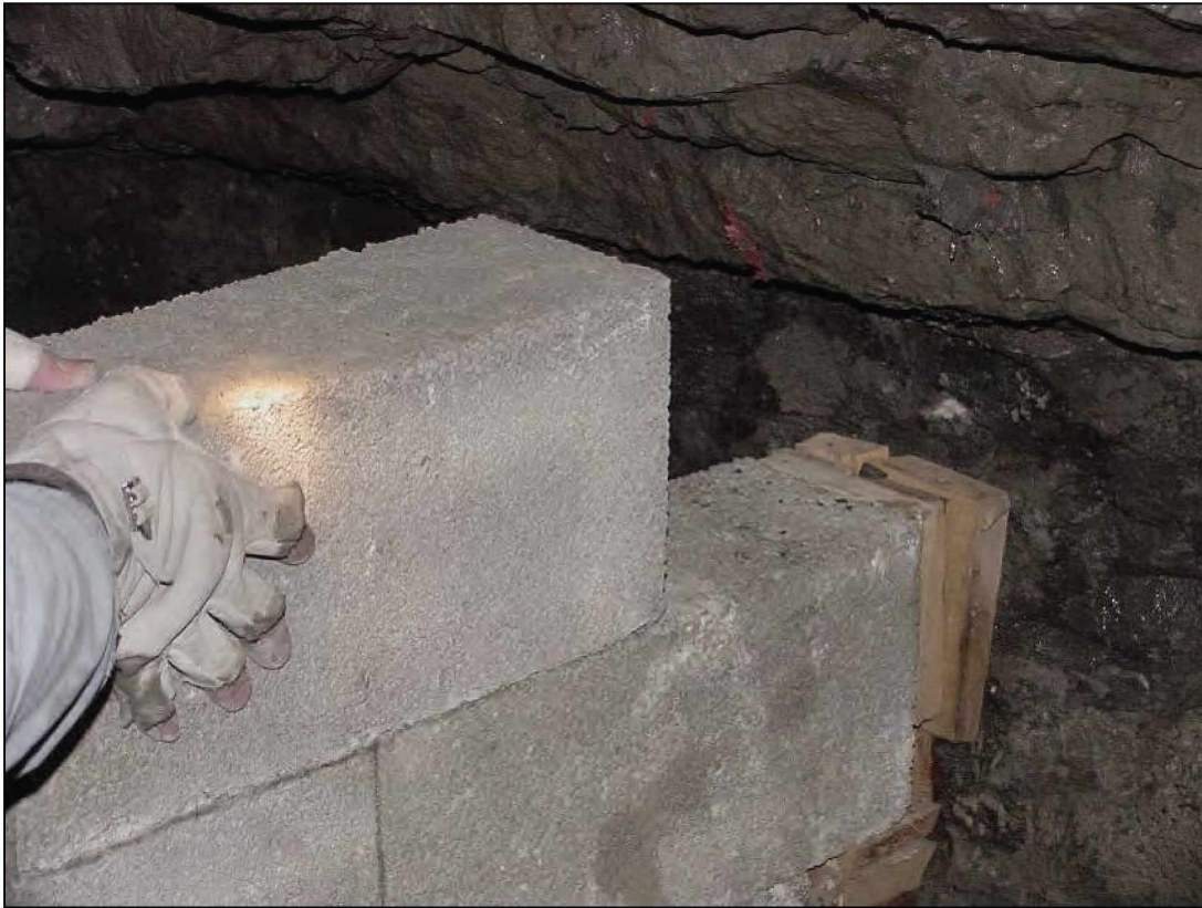
Figure 8.—Dry-stacked solid-concrete-block stopping construction with staggered joints.
