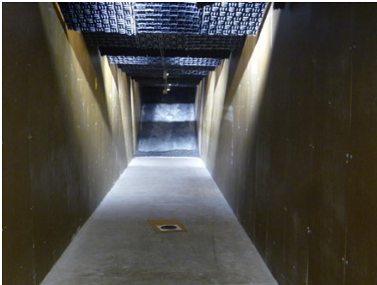
Figure 1. Single lane firing line with rubber tire bullet trap. Photo by NIOSH.
