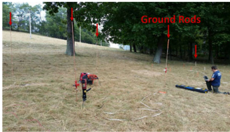
Fig. 10. Testing at one end of an earth electrode.
