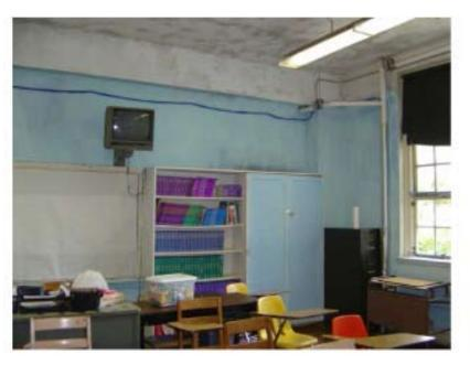
Figure 2. Picture of fourth floor classroom wall and ceiling showing active mold growth at AFSHS
