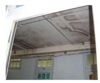
Figure 1. Picture of mold growing along fourth floor hallway cieling at AFSHS
