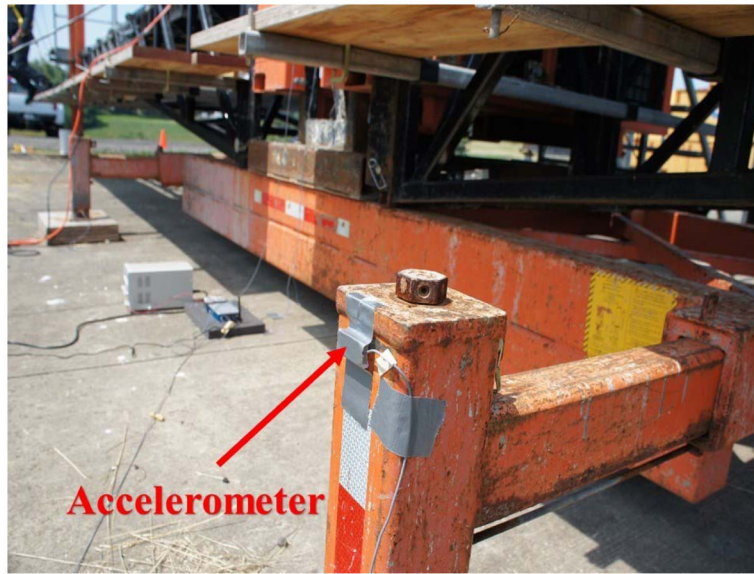
Figure 4. Accelerometer on the outrigger pad column
