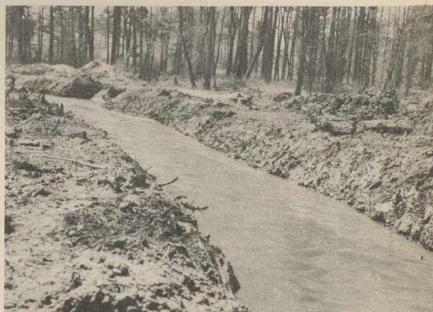
Completed dynamited ditch.
