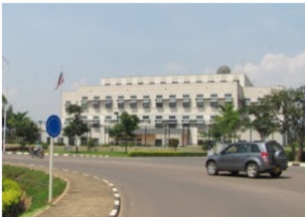
New U.S. Embassy building in Kigali, Rwanda
