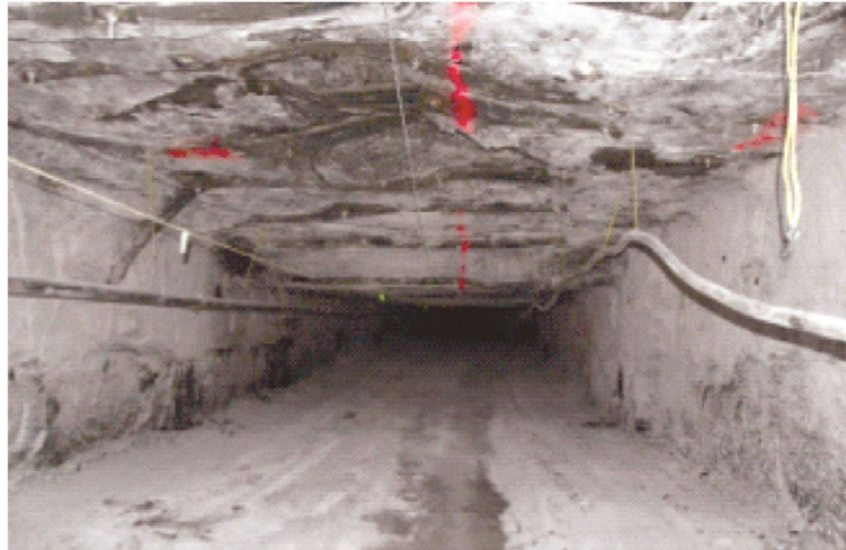
Fig. 3. Entry #4 panel L3 exhibiting good conditions, common to all panels observed.
