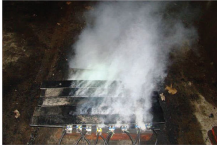
Figure 5. Conveyor belt with electrical heaters beginning to smoke.
