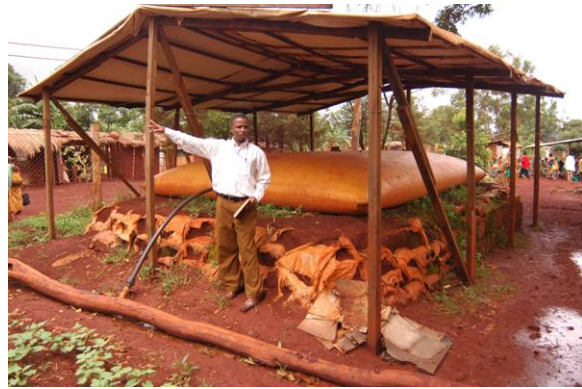
Water storage bladder at Mtabila II Dispensary
