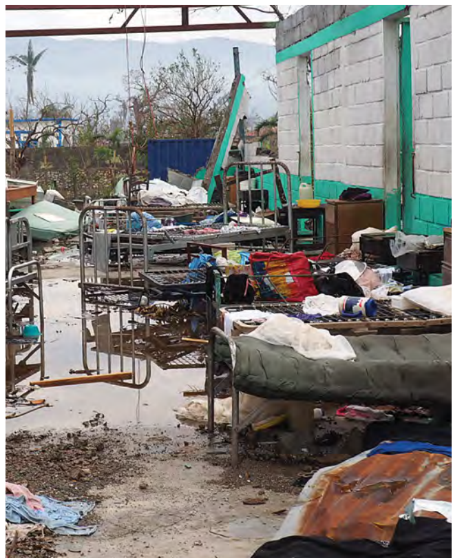
Mental Hospital in Marfranc, Haiti after Hurricane Matthew struck.
