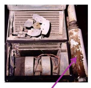
Damaged pre-filter canister
