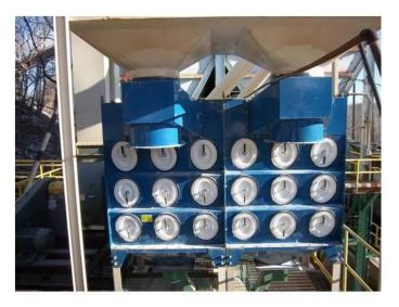
Figure 1.20. Cartridge collector with dust filter canisters.
