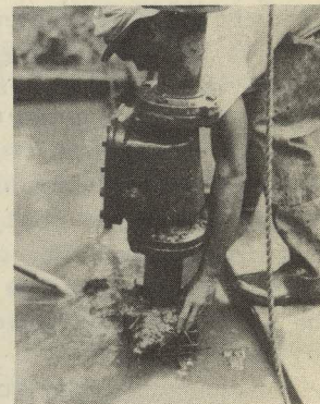
CLEANING TRASH FROM INTAKE
