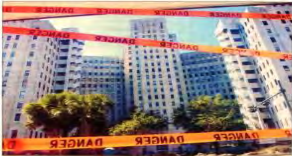
WARNING 1 Caution tape warns people away from Charity Hospital. Damage from Hurricane Katrina has left the hospital unusable, teeming with not only mold but also potentially lethal bacteria. (2005 PHOTO BY NAIT BEAL)
