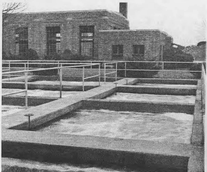
Trainees receive actual field experience in the operation of municipal water treatment plant.
