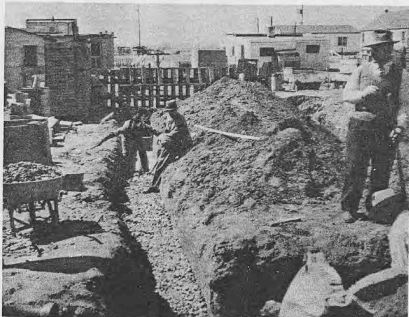
Trainees making actual installation of septic tank and drainage field.
