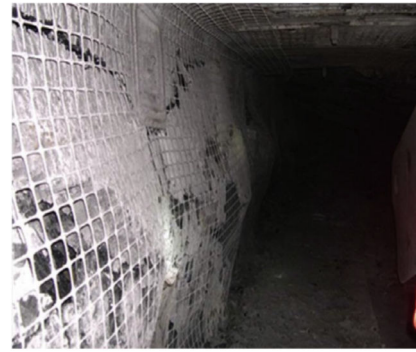
(b) Synthetic grid mesh at the tailgate entry, mine SR 4
