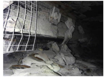
(c) Clay band in the rib at mine SR 5
