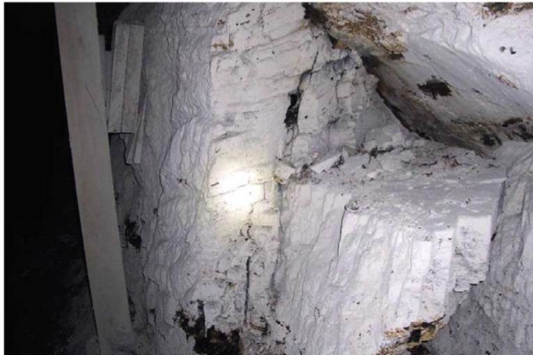
Fig. 16. Large slab formed as result of slickenside plan chuting the rib at mine USR 4.
