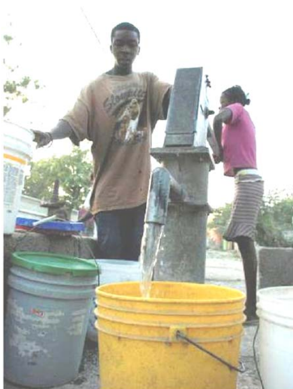
Installation of potable water pumps in public sites
