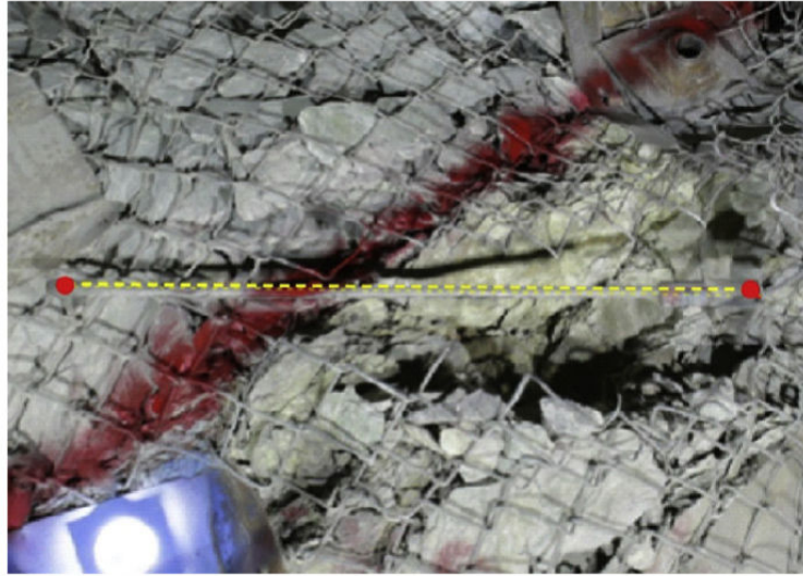
Fig. 9. Crackmeter installation (yellow dotted-line) across fault (red spray paint).
