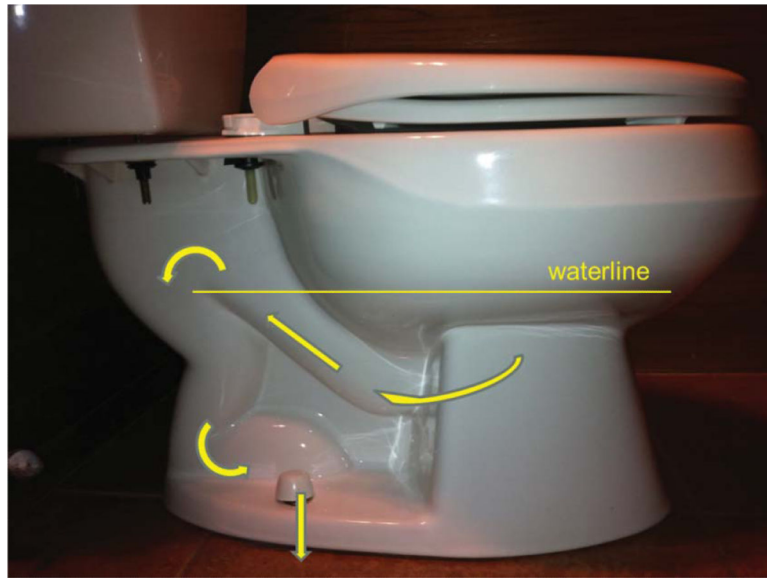
FIG. 2. Typical water flow in the base of a siphonic toilet. (Color figure available online.)
