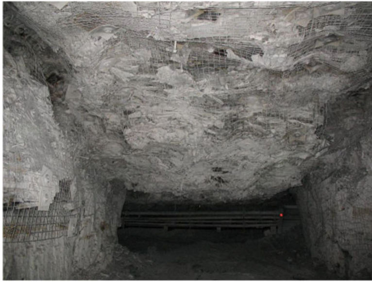
Fig. 13. Example of roof screen used to control deteriorated roof
