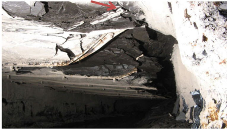
Fig. 7. Buckling of strata associated with cutter formation has defined a vertical discontinuity (seen by the arrow ), which in turn has allowed cantilevering off the opposite rib
