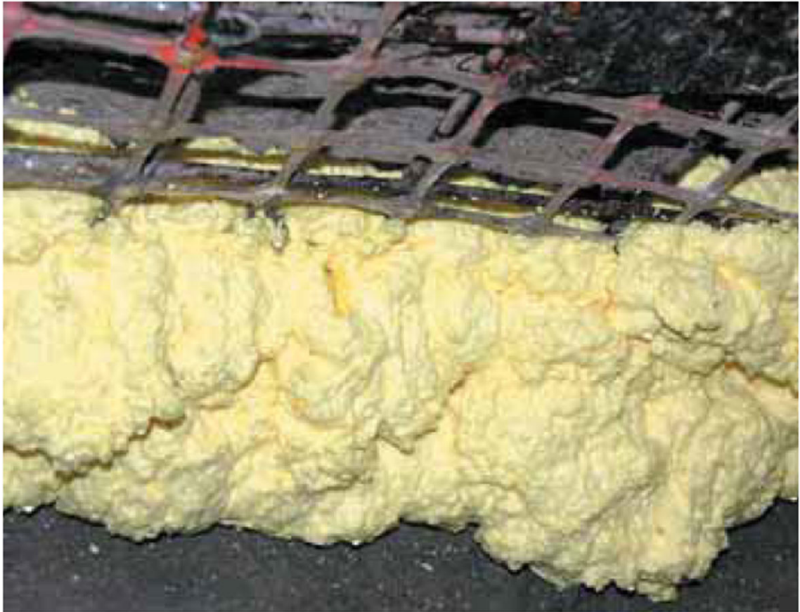
Figure 4. Polyurethane foam sealing stopping at roof on pressurised stopping side for Test 3
