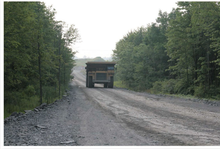
Figure 1. Example of a haul road an operator would travel from the load site to the dump site.
