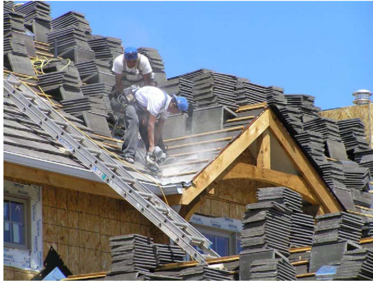
Figure 1. Roof arrangement while installing tiles
