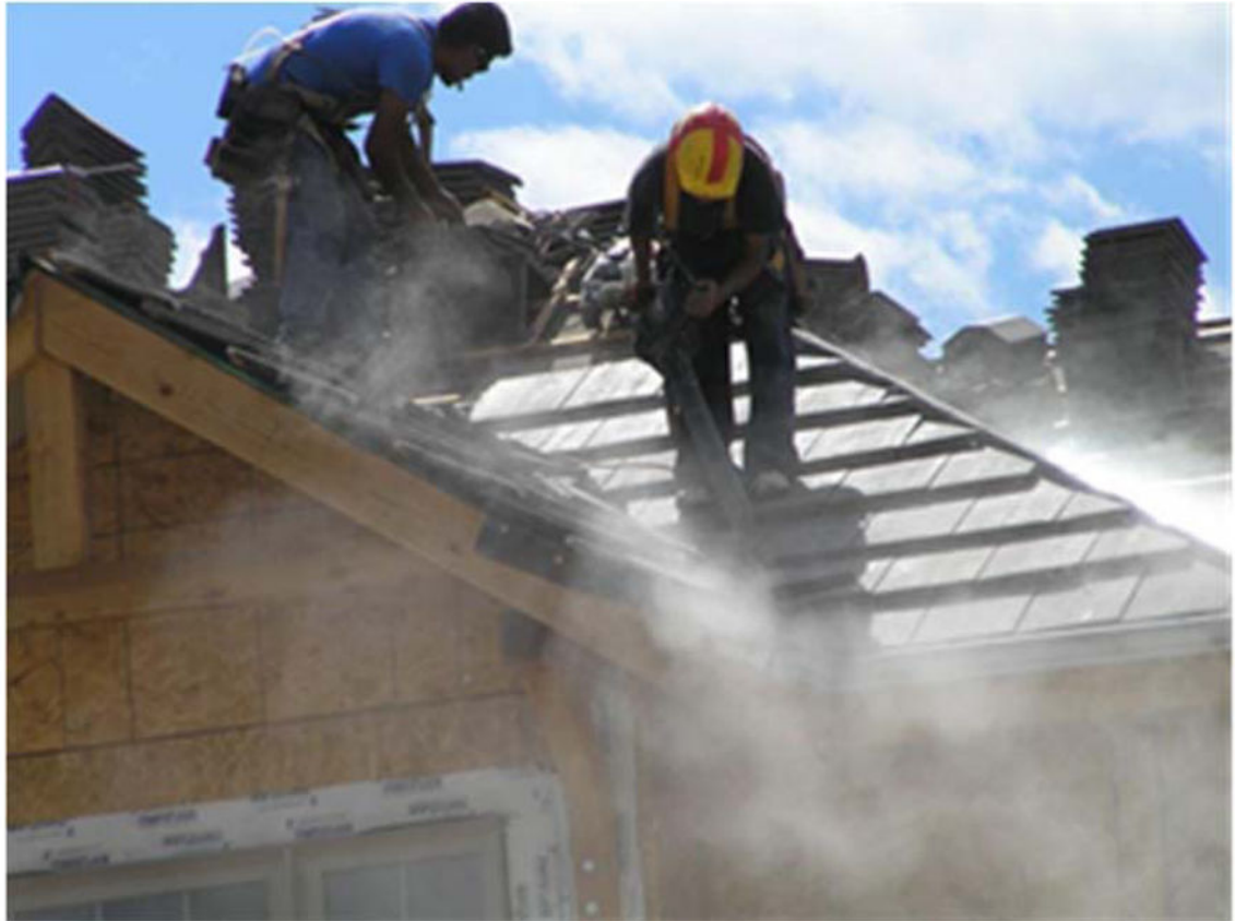
Figure 4. Workers using a leaf blower to clean dust from tiles
