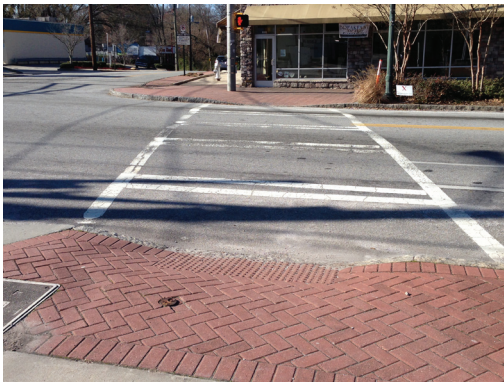
Curb cut (w tactile Paving/truncated dome)
