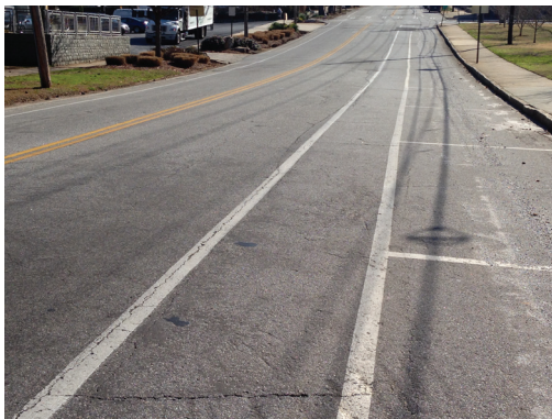
Wide marked bicycle lane
