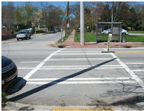
High-visibility striping (Curb cut w/tactile paving, additional crosswalk signage)
