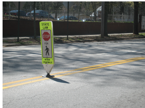
Additional crosswalk signage
