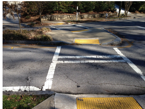
Curb cut (w tactile Paving/truncated dome)
