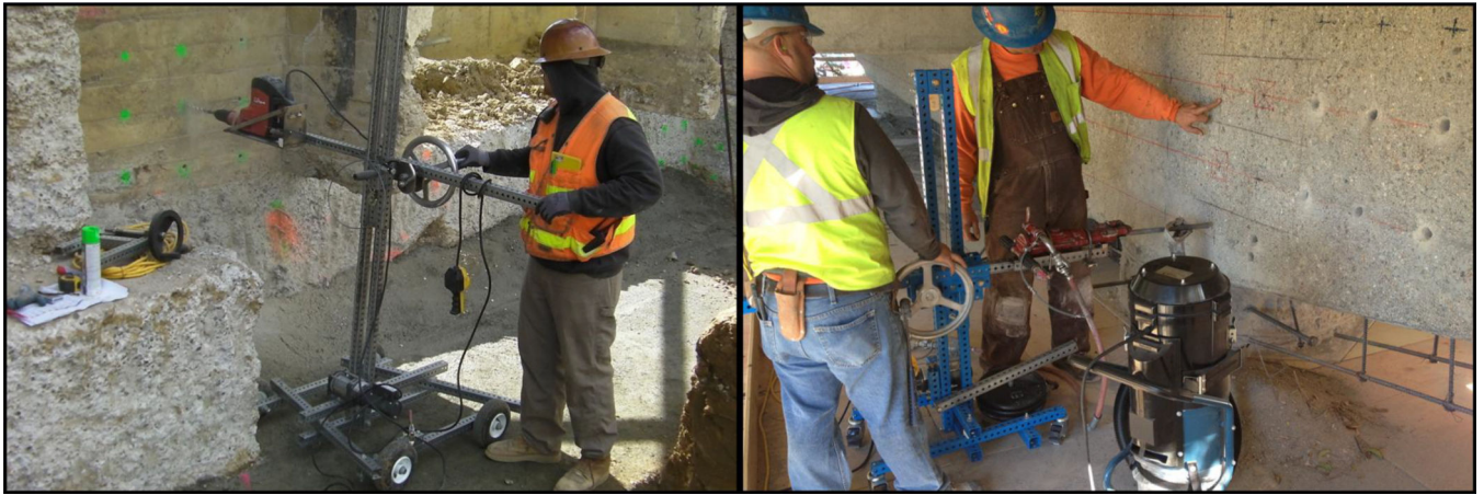
FIGURE 2. Construction workers using the universal rig with an electric hammer drill on a stadium upgrade (left) and a pneumatic rock drill on a train tower (right).
