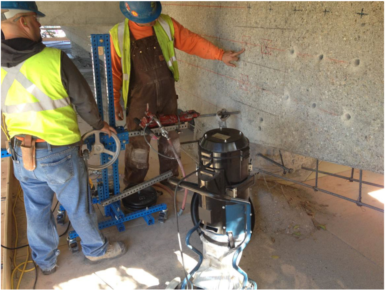
FIGURE 1. Usual method for drilling with a 36 lb pneumatic rock drill to drill hundreds of holes for structural upgrade to concrete columns supporting train tracks.
