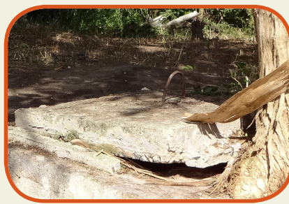
Repair broken septic tank covers
