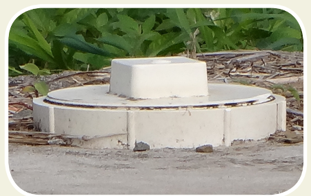
Septic tank sealed with PVC cap
