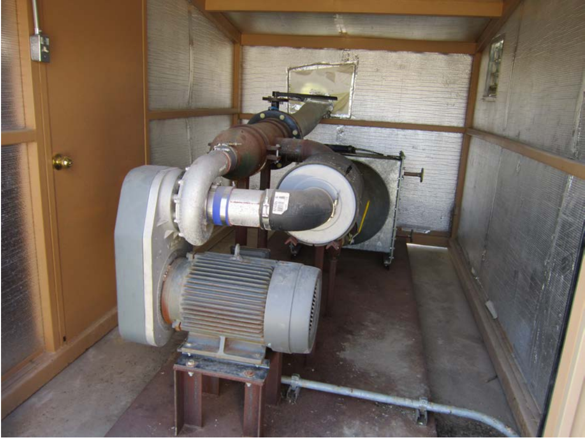
Figure A4. Permanent blower air supply system.
