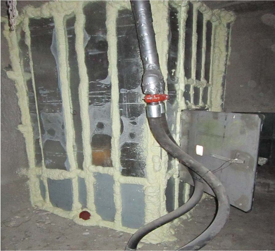
Figure A9: A mine-constructed isolation room for a toilet.
