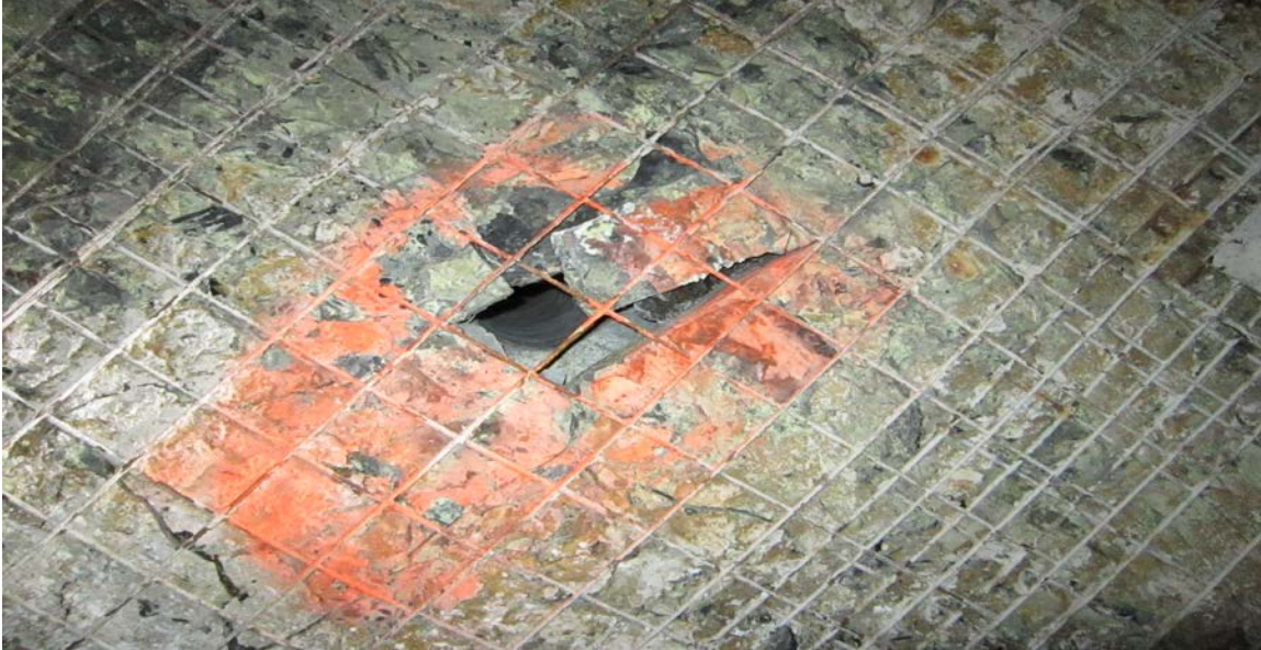
Figure A7. Breathable air supply borehole opening into a built-in-place refuge alternative with no collar.
