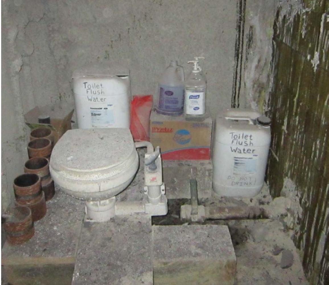
Figure A8: A marine-type flushable toilet.
