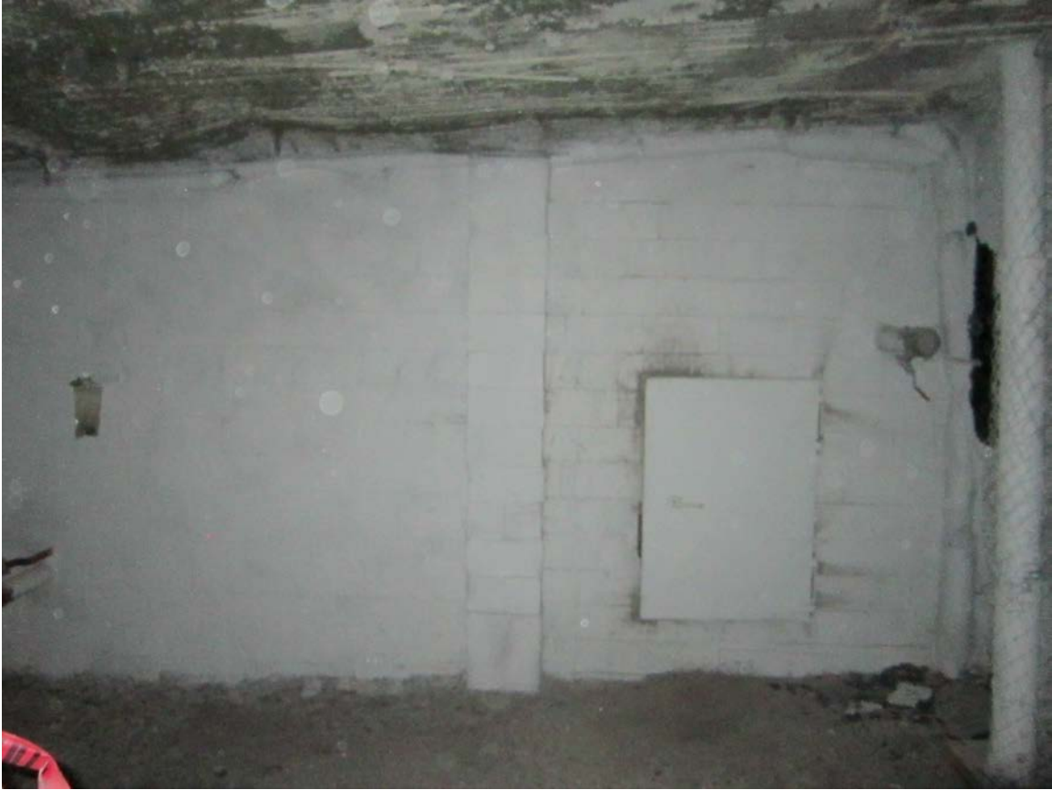
Figure A2. Mine-designed and MSHA District Manager-approved built-in-place refuge alternative stopping and door system.
