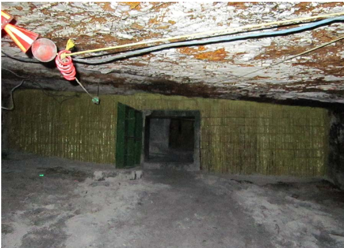
Figure A1. Example of a MICON built-in-place refuge alternative stopping and door system.
