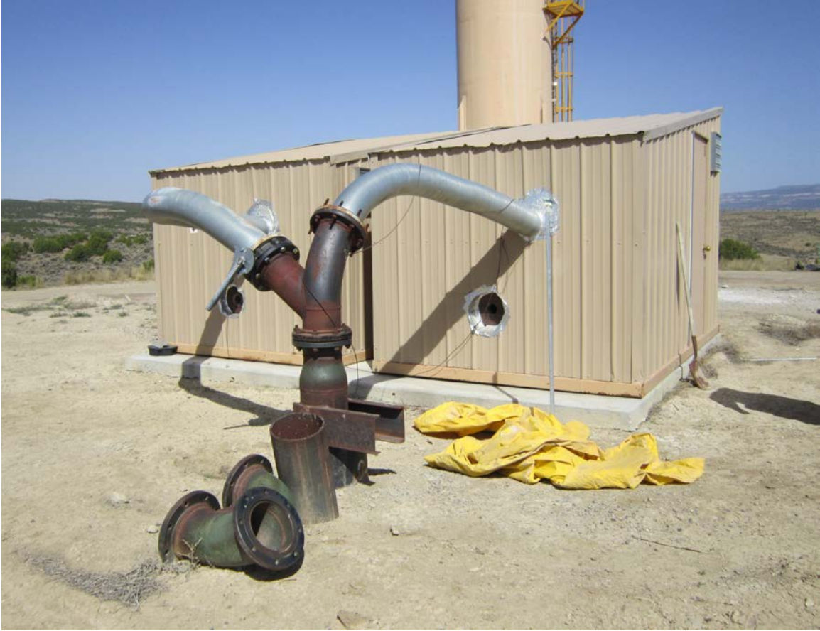
Figure A5. Connection to borehole for a permanent air supply system.
