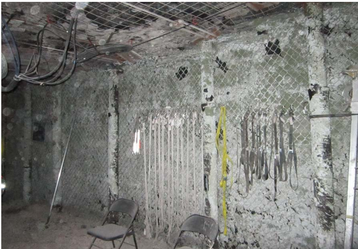
Figure A3. Posts and chain link fence placed to prevent rib rolls in a higher seam built-in-place refuge alternative.
