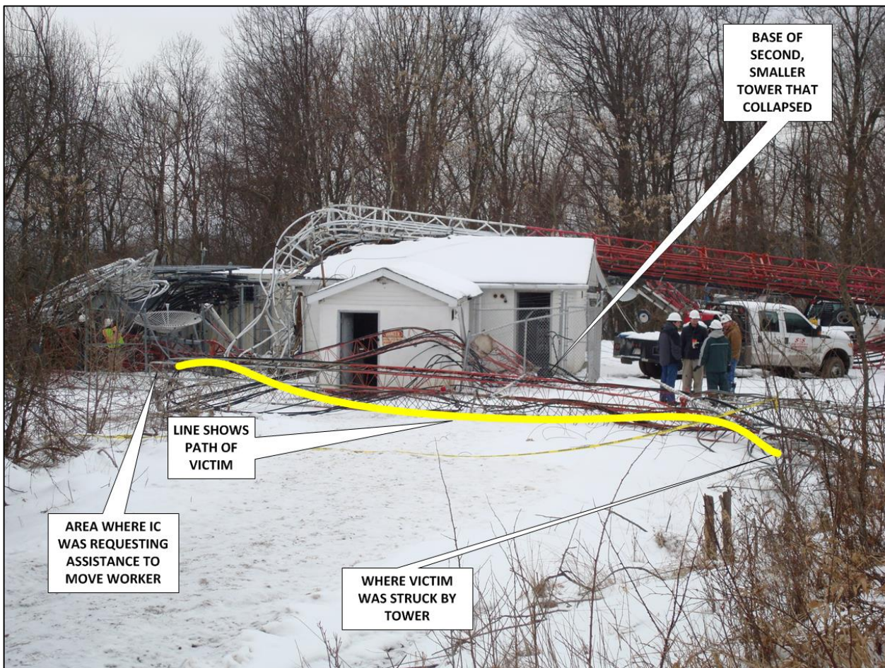
Photo 3. Locations of operations inside danger zone. (Photo NIOSH)
