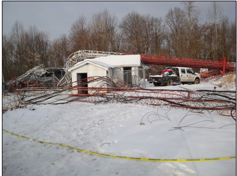
Site of collapsed cell phone towers. (NIOSH photo)
