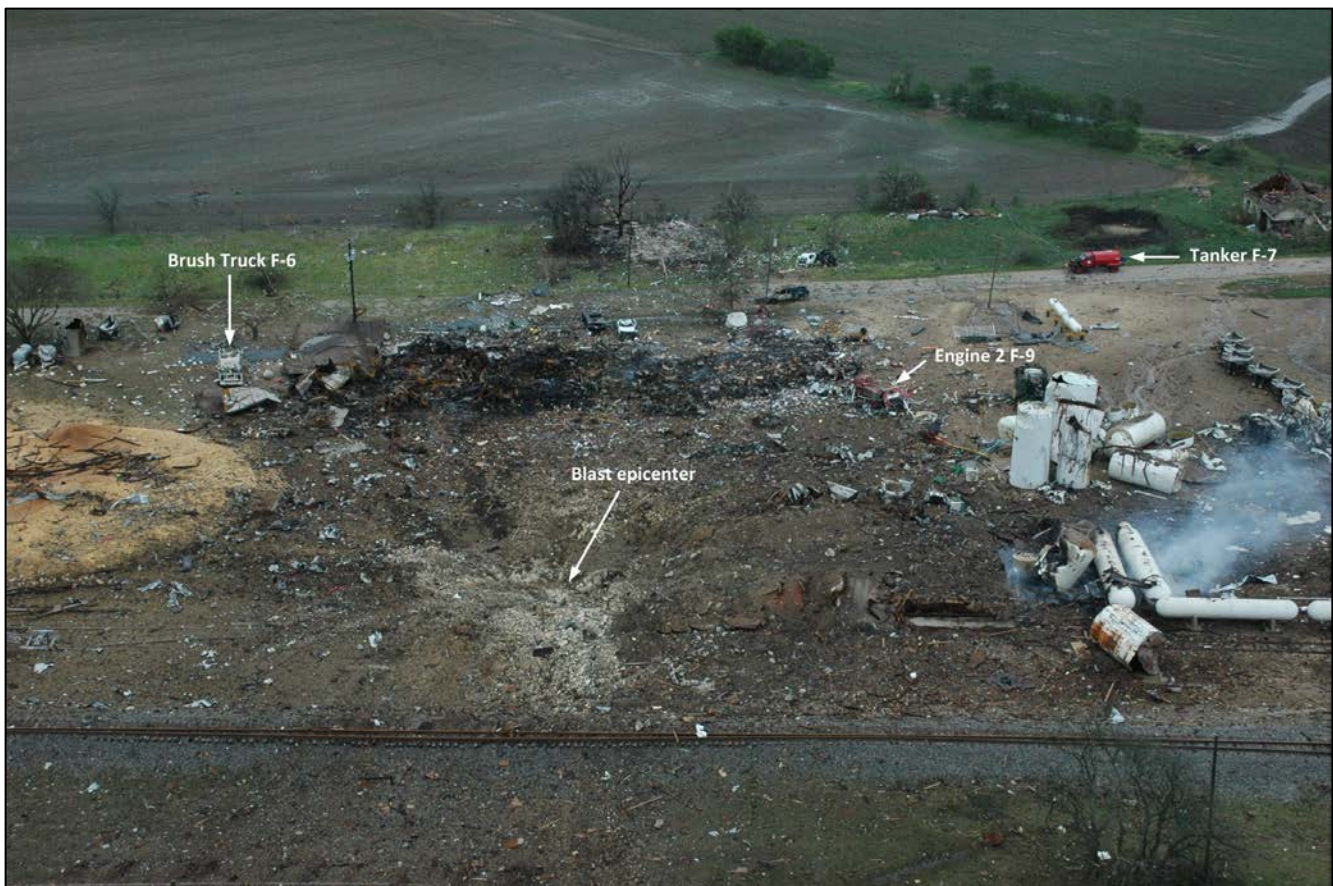
Photo 9. Photo shows fire apparatus locations post-explosion. Orientation is looking east. (Photo source – ATF.)
