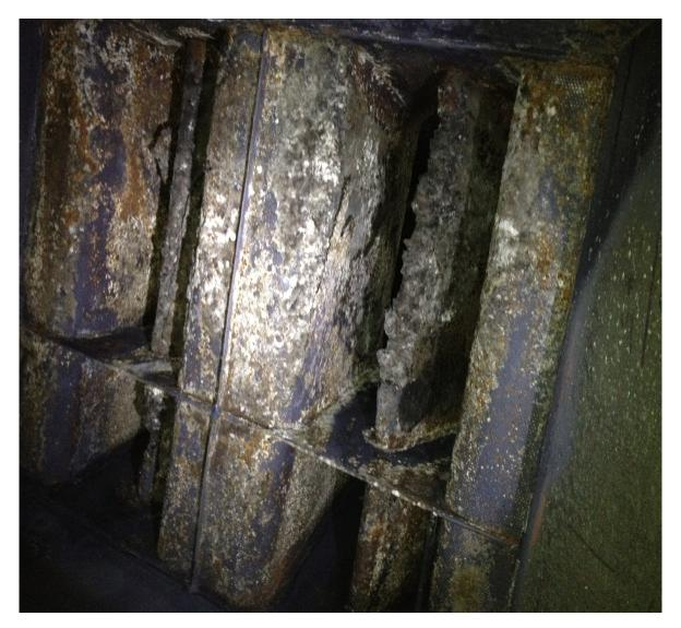
Figure B3. Deteriorating material and mold growth in the 2nd floor HVAC unit ductwork.
