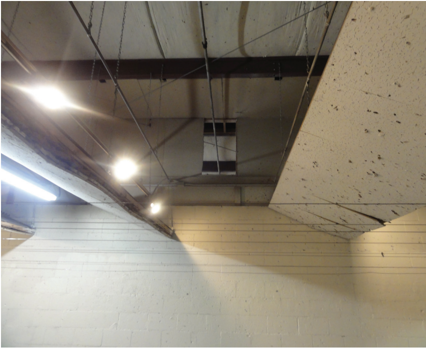
Figure 5. Large hole in the wall that divided ranges A and B. Photo by NIOSH.
