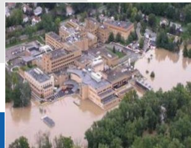
Flooding of Lourdes Hospital, Binghamton NY, 2006
