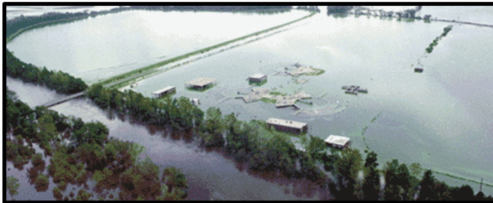
Flooded wastewater treatment plant in Goldsboro, NC (1999)
