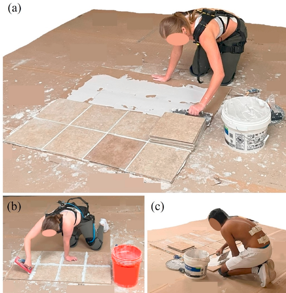
Fig. 1. Illustrations of the tasks simulations: (a) tiling using the HeroWear Apex (HW); (b) grouting using the Laevo Flex (LV); and (c) tiling using No Device (ND).
