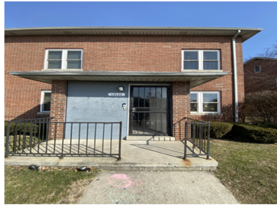
Figure 1. Typical units where energy upgrades were installed.
