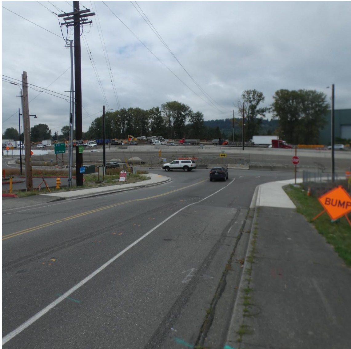
Image 2. Hill where brakes failed with T-shaped intersection at bottom where truck crashed.
