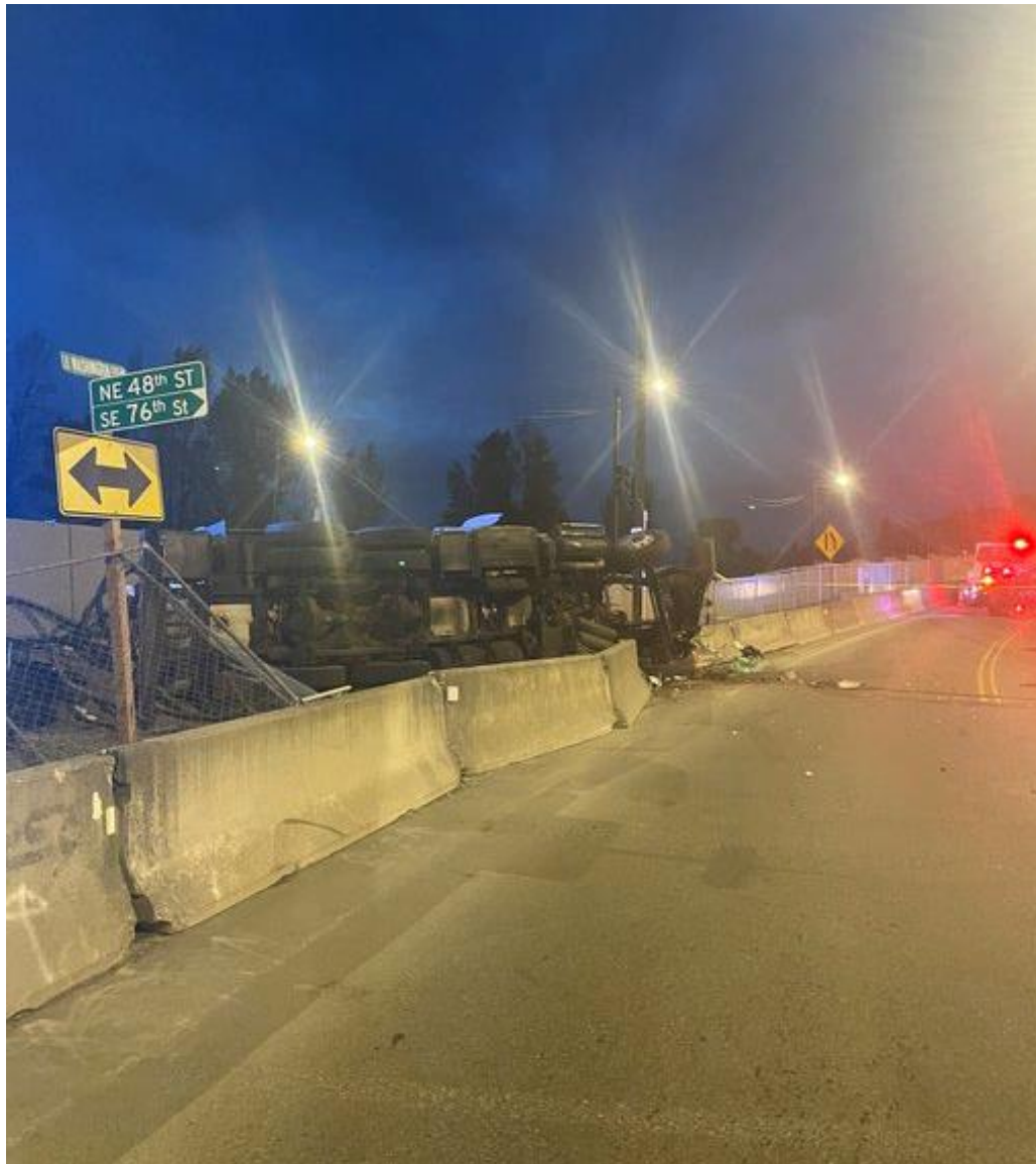
Image 3. Truck resting on side after crashing through Jersey barriers.
