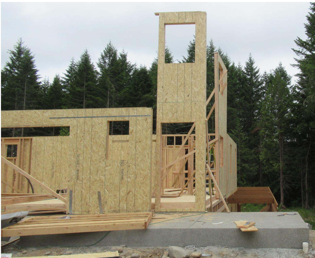
Image 2. Residential home under construction where crew was working.
