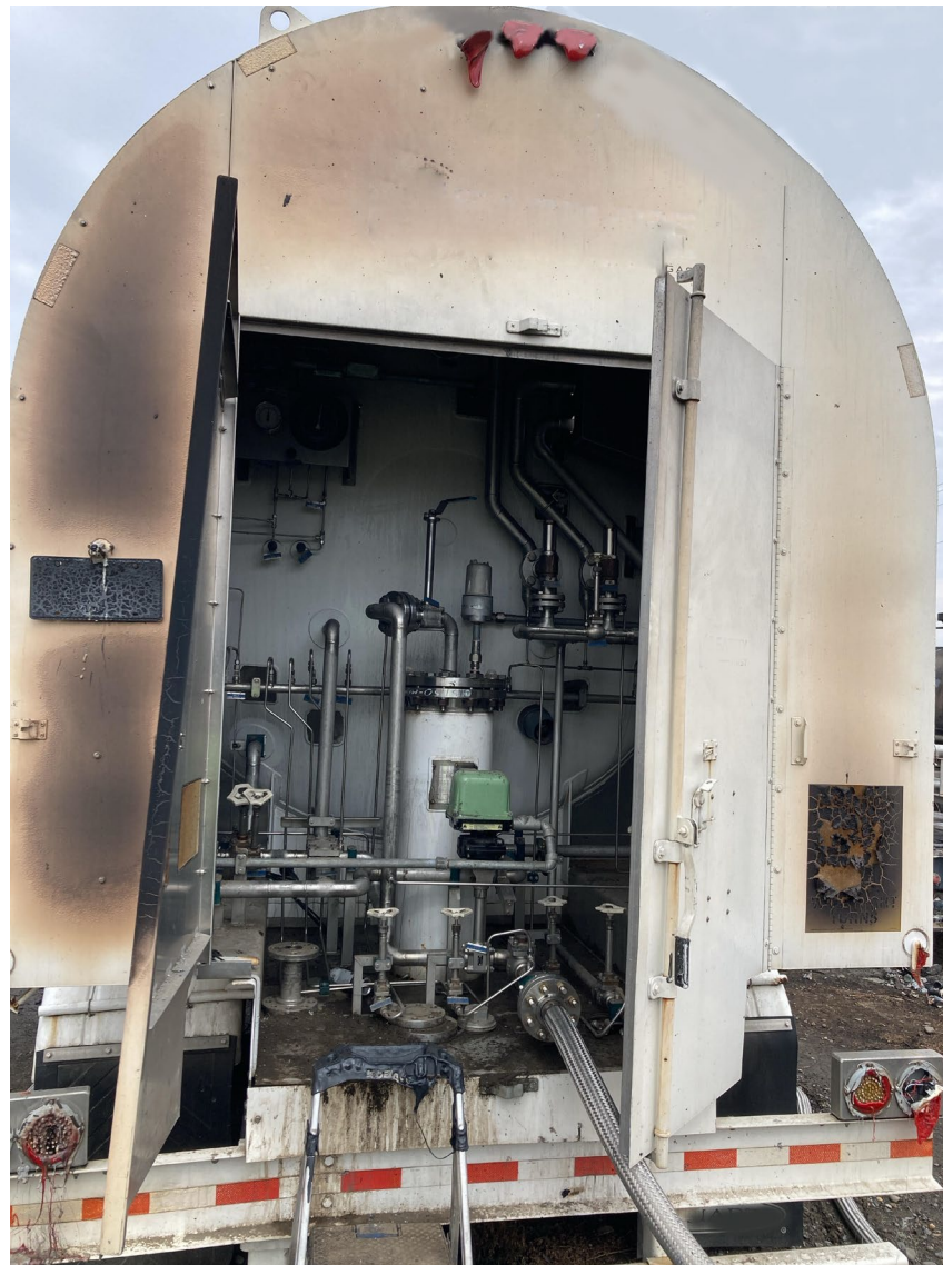
Image 8. Fire damage shown around control cabinet of nearby queen storage trailer.
