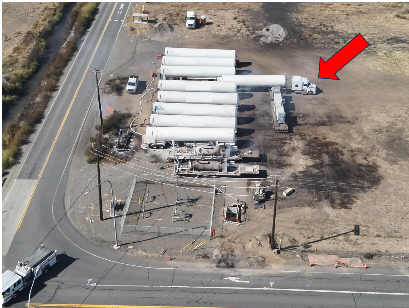
Image 2. Aerial view of LNG transfer station and fire damage to structures and vegetation. Arrow shows truck and transport trailer that pulled forward.
