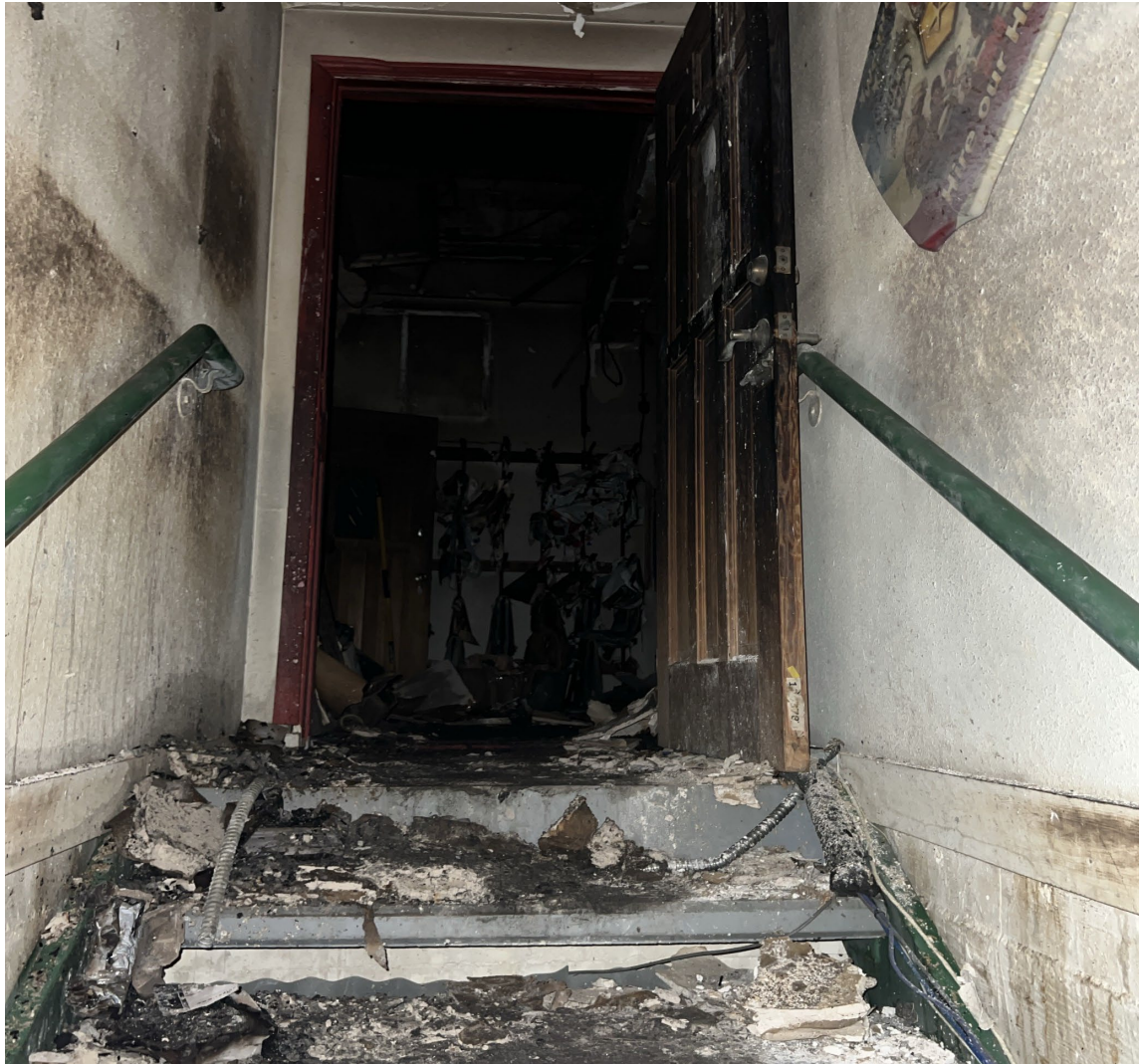
Image 3. Stairway and entrance to second-floor corridor leading to classroom, workshop, lobby, and firing range.
