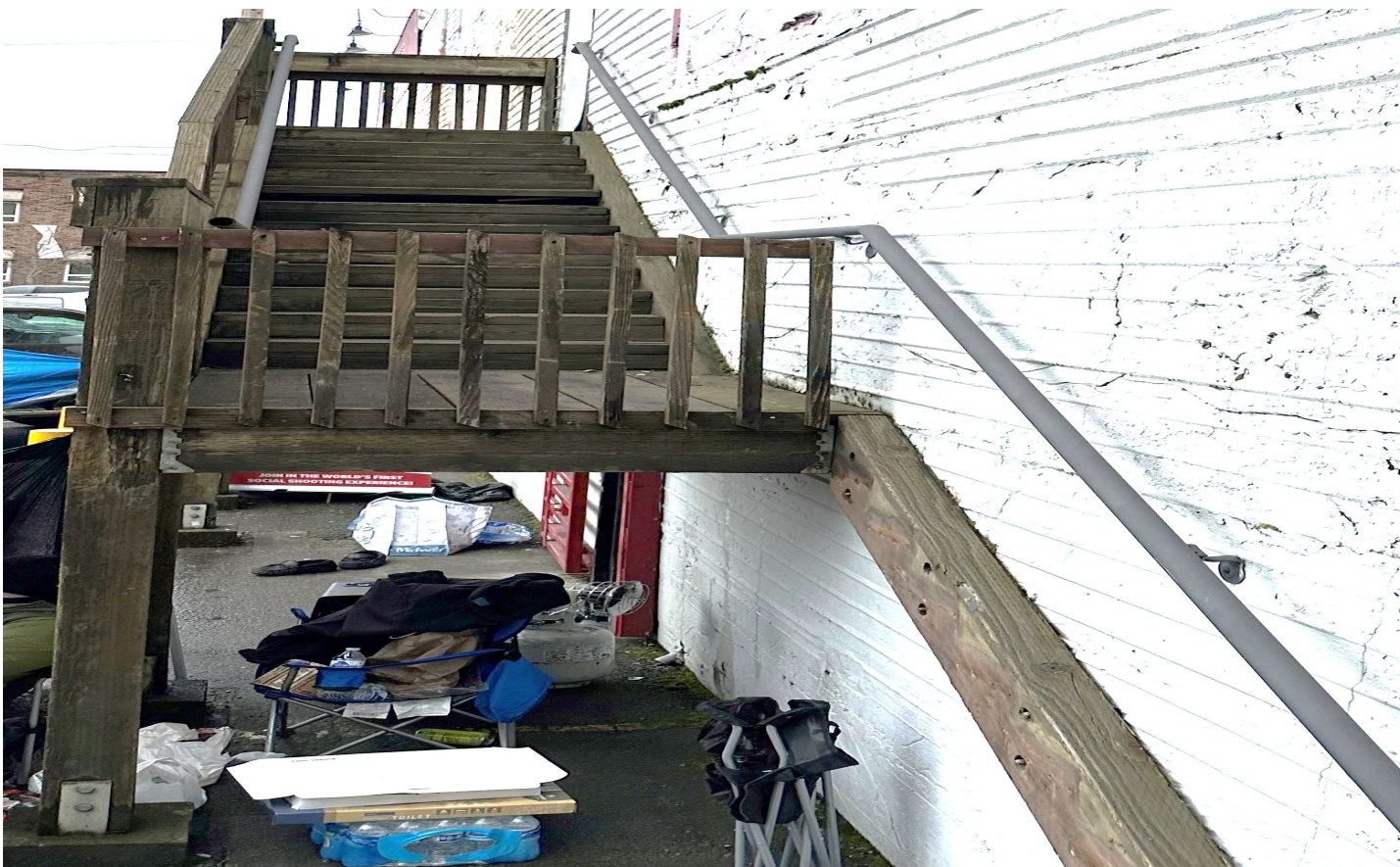
Image 10. Closed external stairway leading from locked second-floor exit door.
