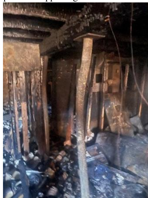
Photo 7: Twisting of steel column. (Courtesy of the fire department)
