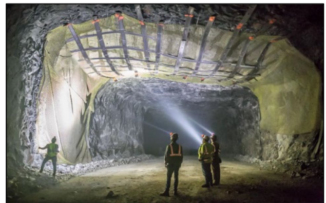
Fig. 4 Ground support around Pillar-X (Credits: R. Bishop)
