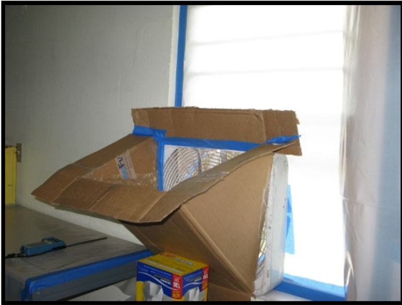
Figure 3. Photograph of Makeshift Hood for Exhaust Fan.
