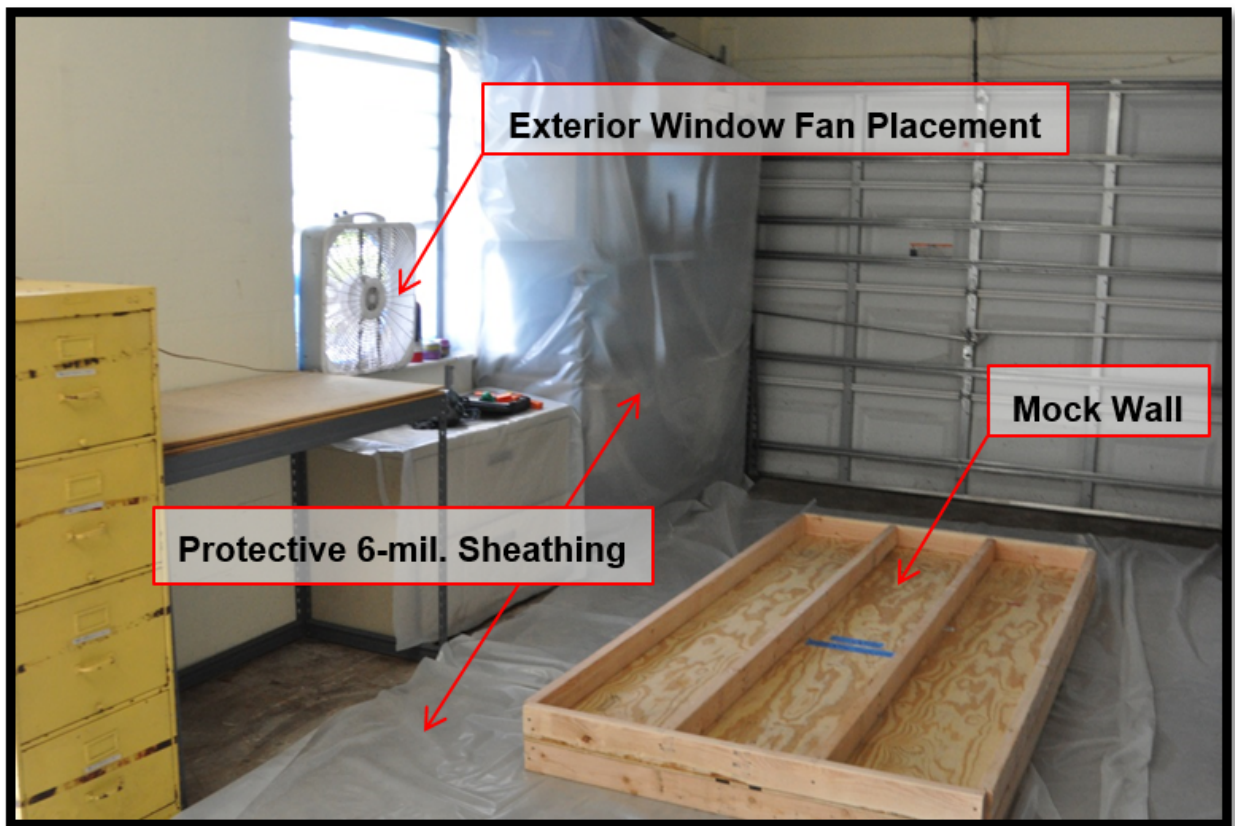
Figure 1. Photograph of Initial Layout of Work Area.
