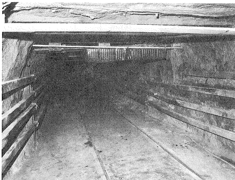
FIGURE 11. - Two PVC water tubs mounted near mine roof.
