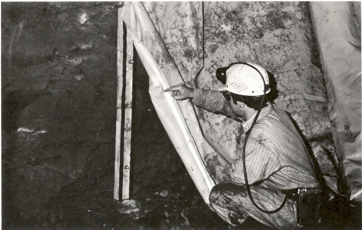
FIGURE 5. - End panel being attached to wall with Velcro seal.
