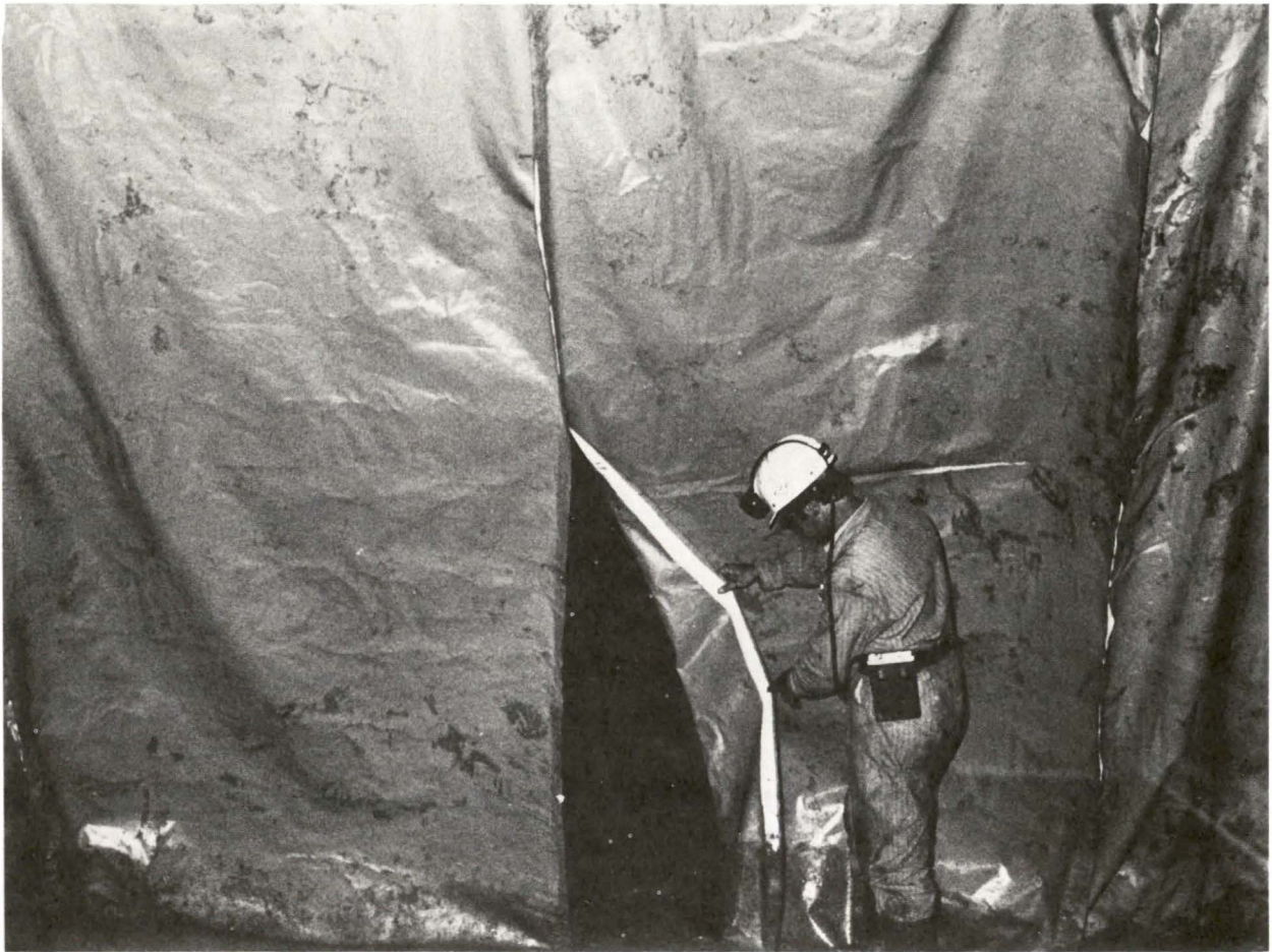
FIGURE 8. - Brattice peeled open by blast.
